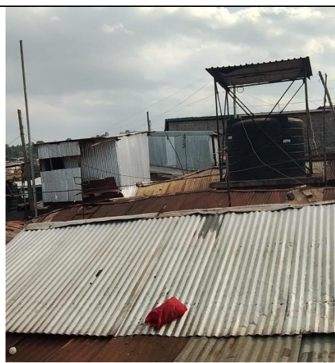
Example of an iron roof and water tank
